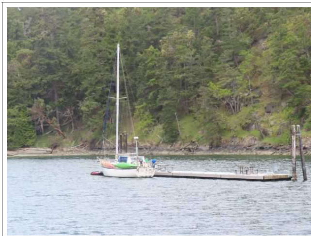
Reid Harbor Floating Dock
