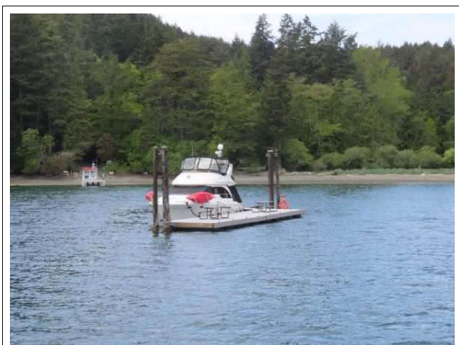
Reid Harbor Floating Dock
